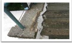
**The solution:** In January 2015, **APA** undertook a series of concrete defect surveys and testing to four reinforced concrete staircases, consisting of visual defect surveys, hammer surveys, cover surveys, carbonation testing and chloride profiling, with the aim of establishing the extent of the repairs required. The solution consisted of the removal of all delaminated, weak, damaged and
